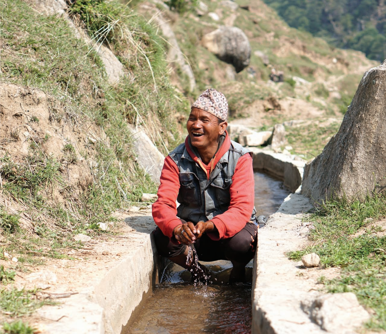
Farmer at irrigation canal built in Jumla in 2018.
