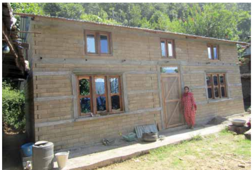
Compressed Stabilized Earthen Brick (CSEB) produced locally and used to construct houses by villagers in Thokarpa, Sindhupalchowk.
