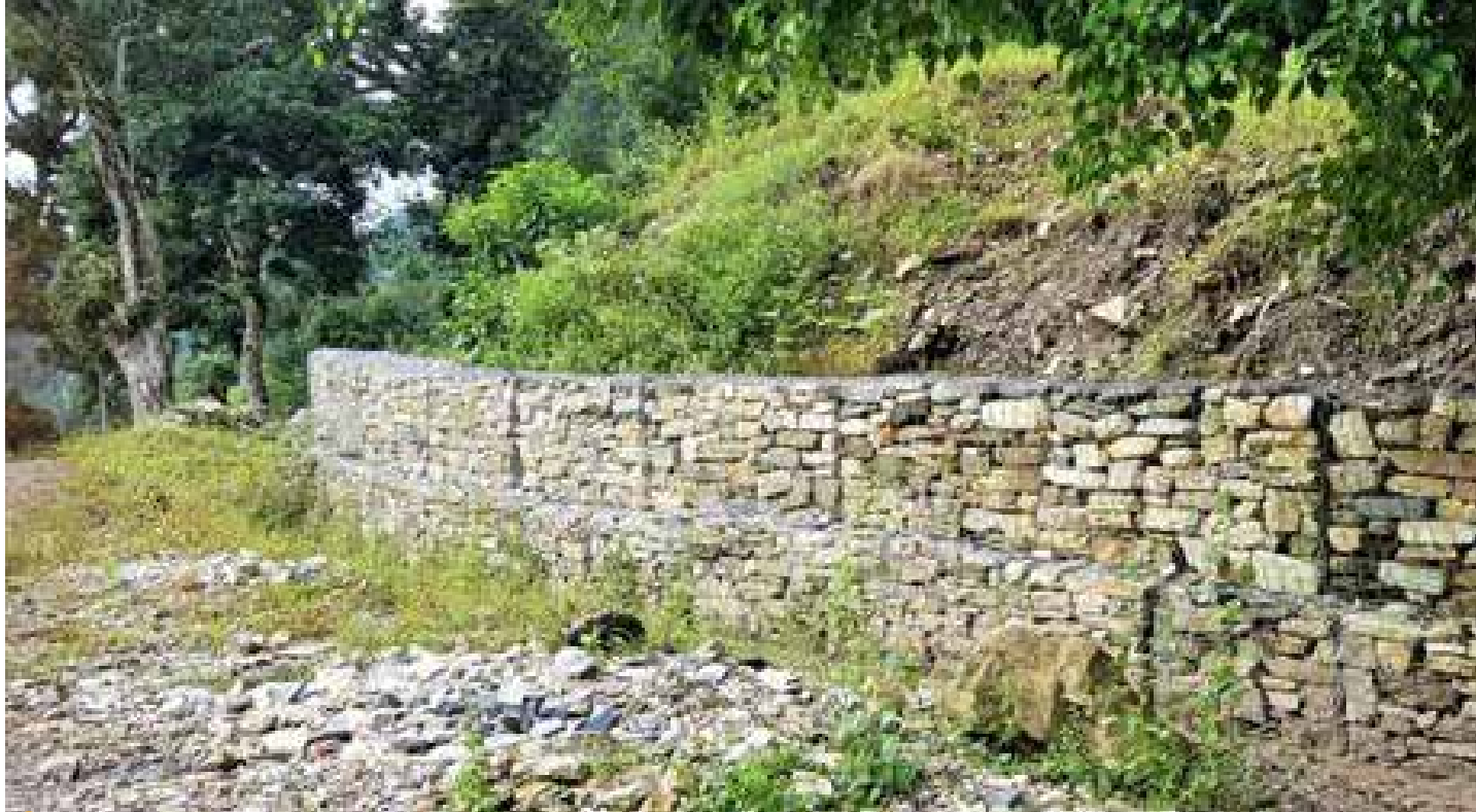
Gabion wall construction to control landslide in Sera, Batase, Chautara-Sangachokgadhi Municipality.
